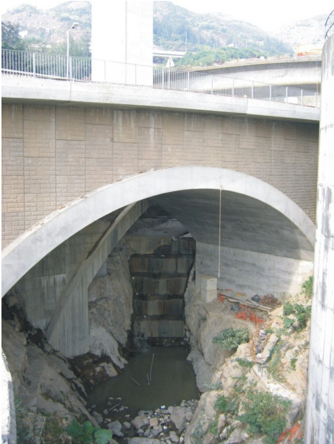
Figure 10 - View of completed arch.
